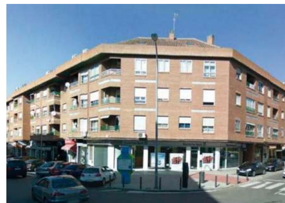
Barrio Sta. Teresa Buildings | Toledo
